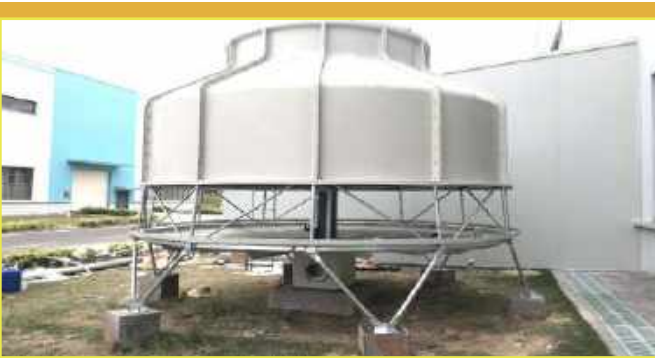
◆ Cooling Water Tower
